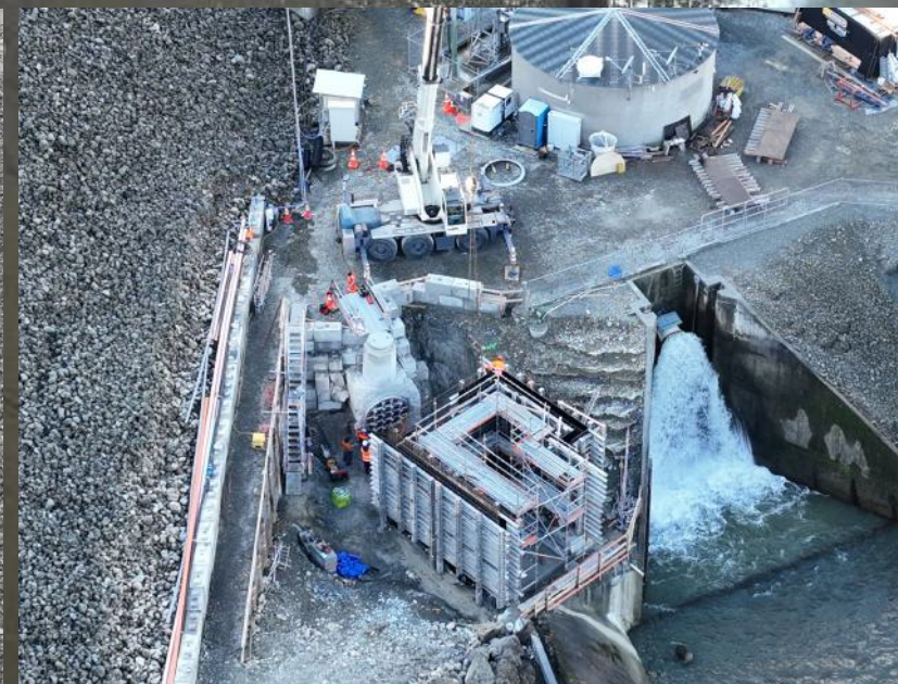
Image bottom right: New flange fitted on the original diversion conduit, form work in place on the valve chamber (August 2024)
