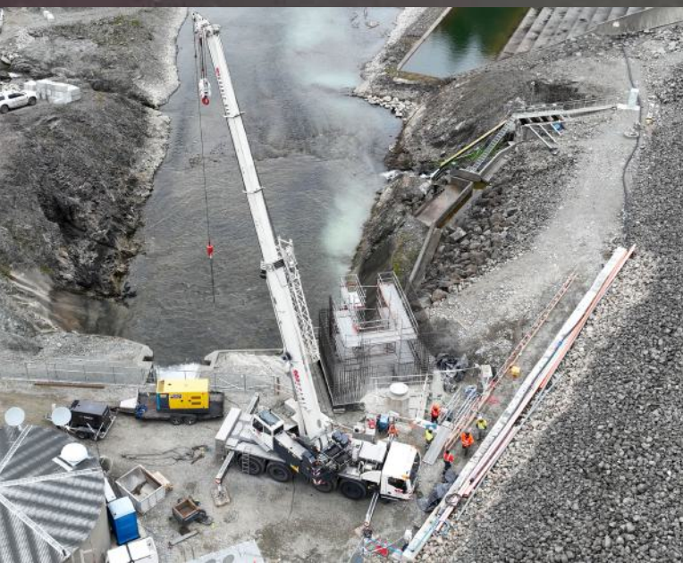
Image bottom left: New valve chamber in construction (July 2024)
