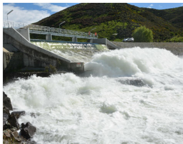
Above: water flowing from Lake Opuha
