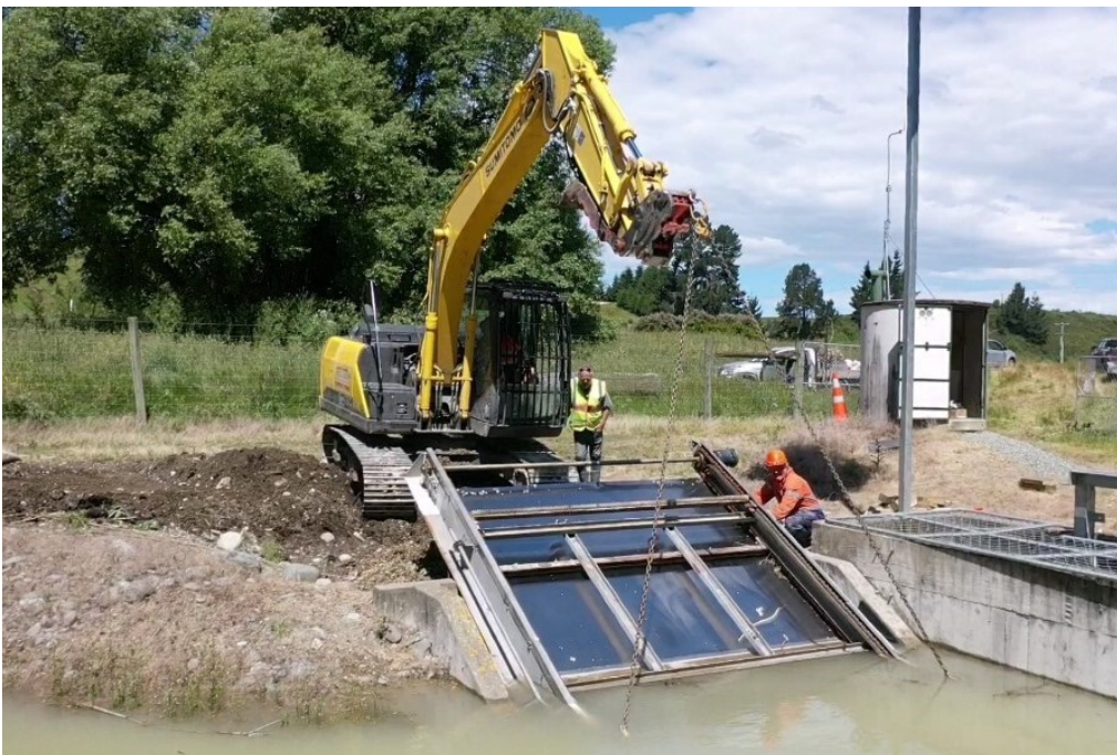
Image of the operations team removing the Skipton screen
