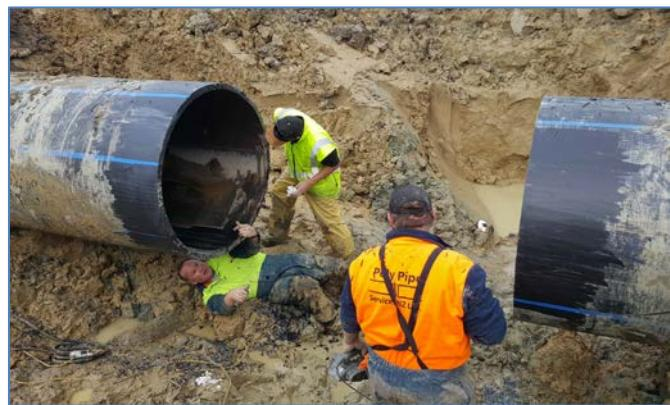
As well as the scheme intakes, there has been some substantial work done on the Kakahu MR1 pipeline to repair some leaking sections. Very challenging work in the wet
